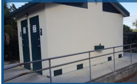
Flood Vents on a Park Restroom
